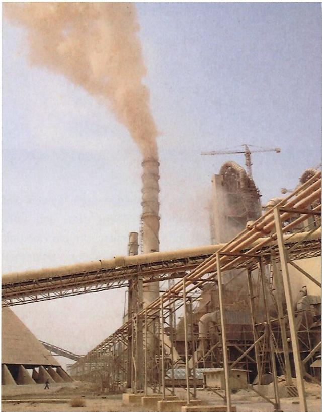
Figure 6: Broken bag filter, which can be monitored and recorded
