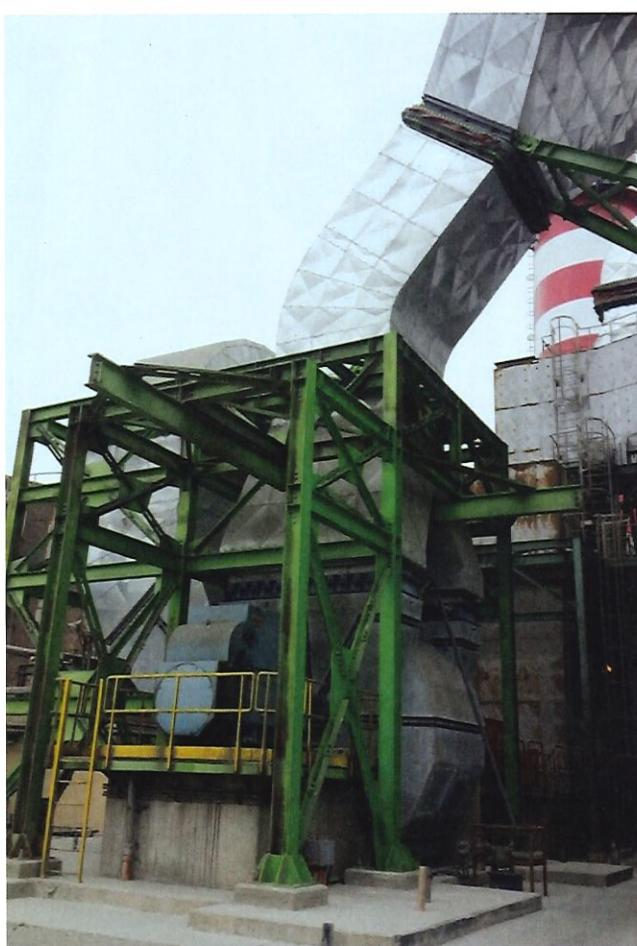
Figure 4: Combination of the process fan and de-dusting filter
